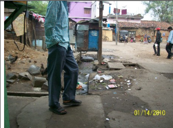
Open Drain Charbhathi Slum
