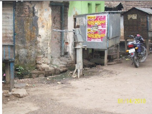
Tubewell without washing platform
